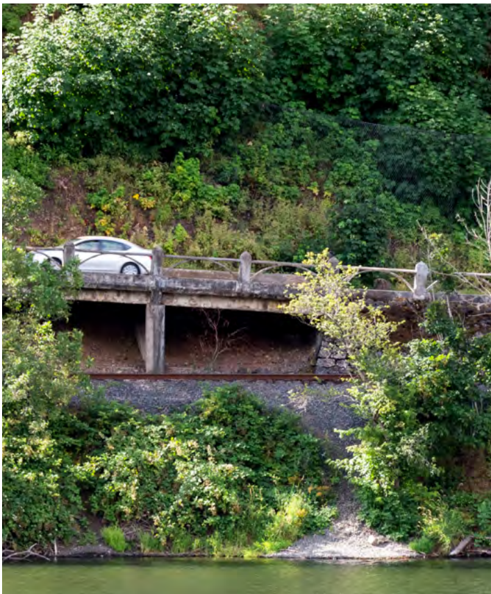
Current photo of the west viaduct near rail line.
